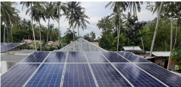
White Trees, 15 KW,p + batteries Lombok
