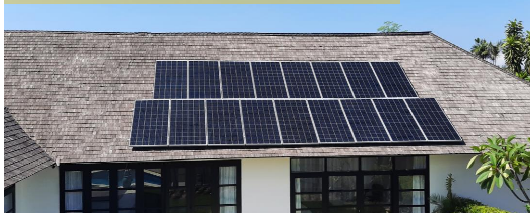
Samara Office, 8kWp + 11kWh batt + Ctrls, Sanur Bali
