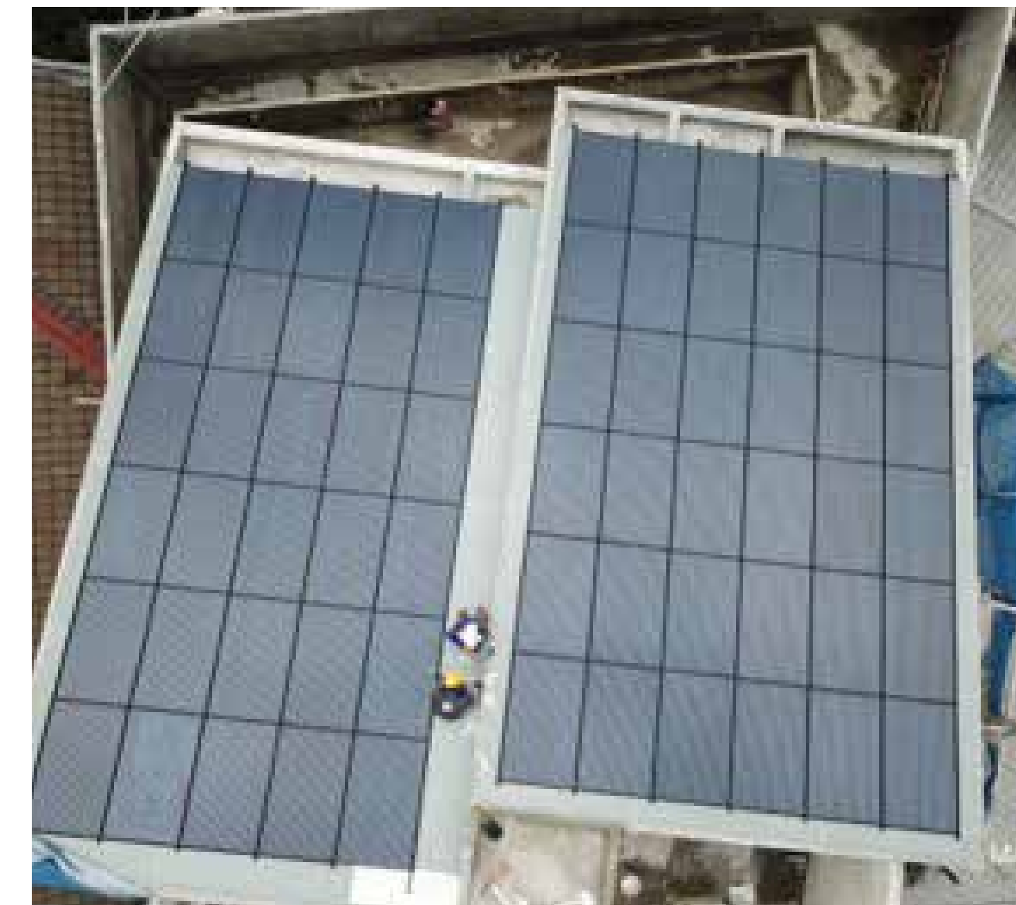
Senopati, Jakarta Residential “SunRoof” 18kWp roof-integrated complete with insulation
